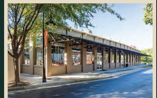
PURITAN MILL ATLANTA, GA 125,000 SF / CREATIVE OFFICE
