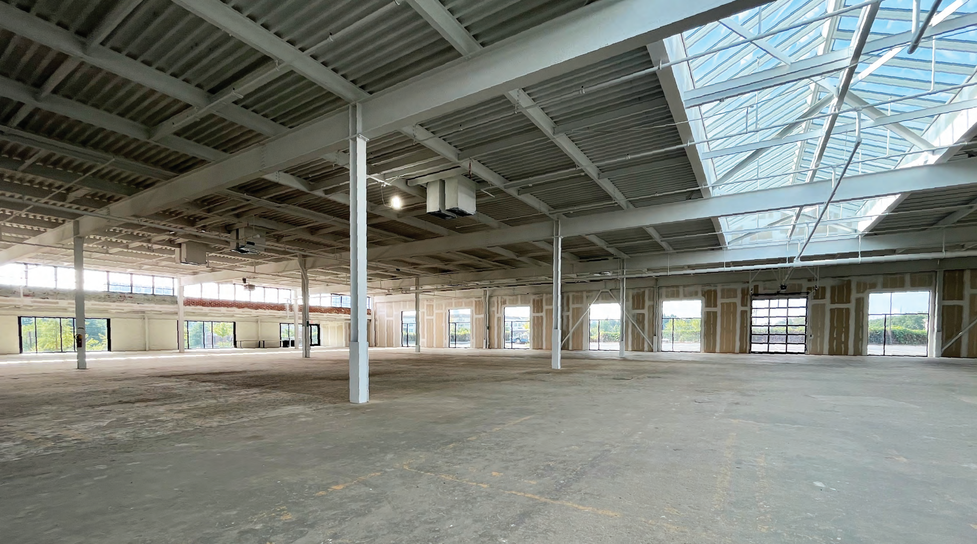
SOUTH BUILDING INTERIOR AND LOADING DOORS
